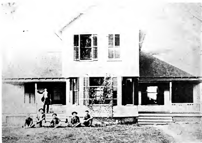
Locktender's house at Lock 19 immediately south of Wyanet. (Photograph courtesy of Hennepin Canal Parkway.)
